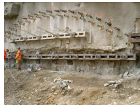
Soil nailing Blanka tunnel Czech Republic
