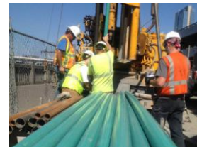
Inclinometer log cases Seattle, USA
