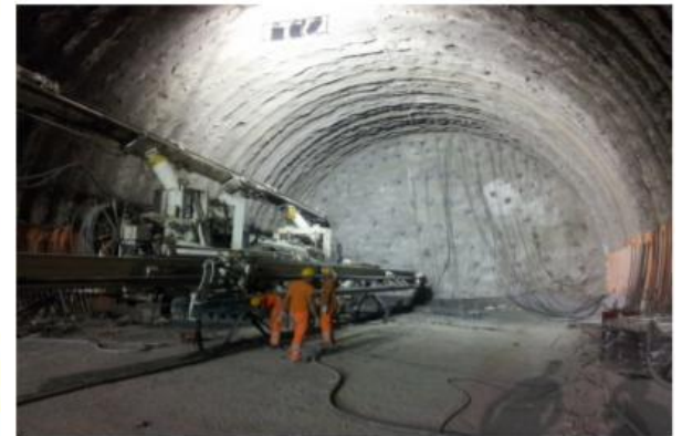
Tunnel excavation for highway construction (GUI)
