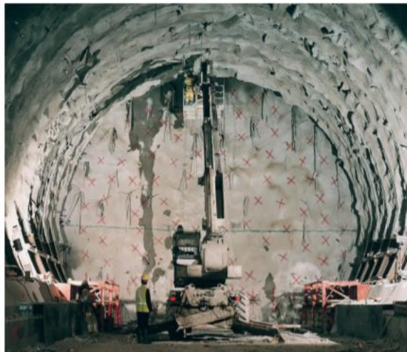
Pre-confinement of excavation front with Durglass GFRP structural elements
