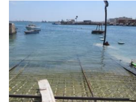
Underwater slab harbor, Italy
