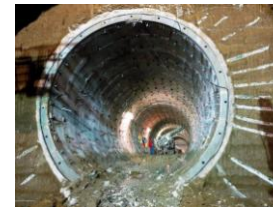
Soil consolidation Duomo station Napoli, Italy
