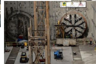
Soil nailing University Link railway Seattle, USA
